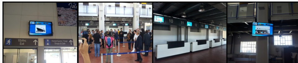
Digital signage installation at the Port of Piraeus
